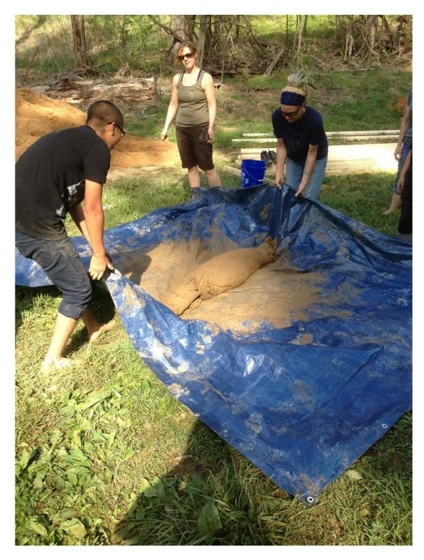
8. Stomp on top of the burrito of cob mixture until its flattened again. Take some handfuls of straw and sprinkle it over the flattened mix. Again start to stomp the cob mixture until all of the straw has been covered and smeared with cob. Use the tarp to gather the mix up and turn it over again. Stomp
