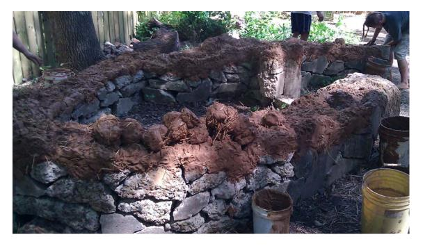
The first part of building your cob home will be the foundation. The foundation holds the weight of your walls, roof, and upper floors. Your foundation will distribute the weight of the house over a large area and prevents it from sinking into the ground, which can be catastrophic to a building's structure.
