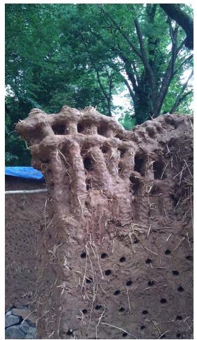
When you place lintels above your openings, make sure to insert temporary supports below them and keep them there until the cob above is completely dried through and solid.
