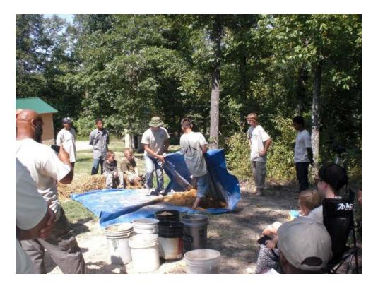
The most basic and one of the most practical ways of making cob is using the tarp method, which was developed in 1994 by a cobber in North America named Becky Bee.
