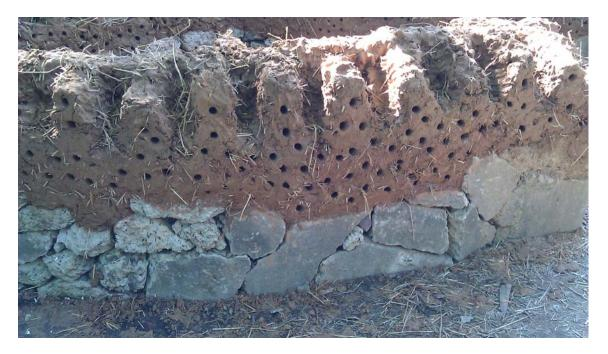
When you're done with a layer of cob or if you're finishing up building for the day, make a spine and ribs. Make a ridge of cob loaves down the center of your wall, attached well together and attached well to the bottom. On both sides of the ridge attach cob to it at right angles going from the ridge to the edge of the wall on the inside and outside. Between each rib, just leave about the space of one cob loaf. These gaps will be filled in first when you start the next layer.
