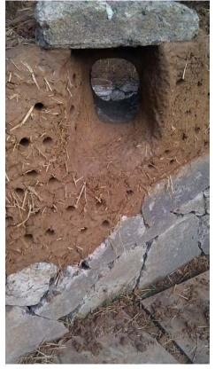
glass. Your glass and padding can sit on top of the sill. Make your window sill on the outside slope downward away from your window. Your sills can be made of various
