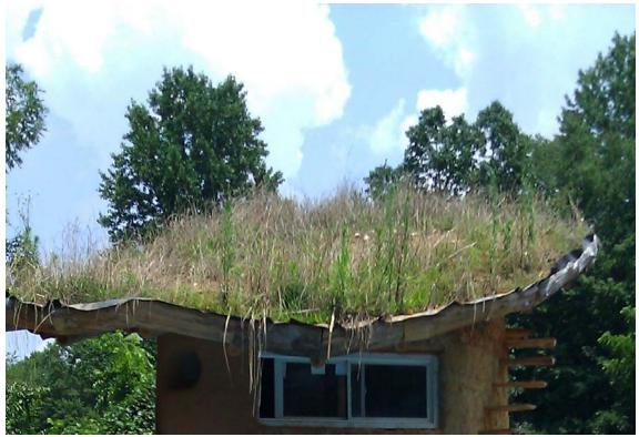
Natural builders are always interested in how to construct living roofs. They complement cob and natural building very well and are very economical. A living roof is basically a roof that has a layer of soil and vegetation growing in it. Sometimes they are called sod roofs. This kind of roof is becoming more and more popular these days and can even be found in cities on top of large buildings.
