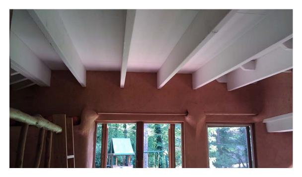
Your indoor ceiling acts as a support for your roofing insulation and provides an attractive surface. There are a lot of ways to do a ceiling. You can put the ceiling in strips between rafters, beneath rafters, on top of rafters (so the rafters still show), between trusses, or suspended down from rafters for more insulation.
