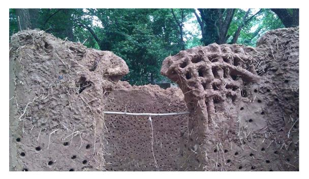
To make corbel cobs you need a wetter cob mix and long pieces of straw. Make your cob mix without putting in the straw. Then take a handful of it and wrap it over a small handful of straw lengthwise to create your corbel "burrito" shape. Knead the cob with the straw so that its all held together well.
